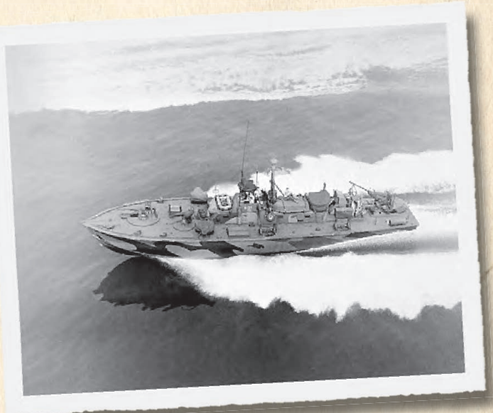
The Navy's Patrol Torpedo (PT) boats were the primary vessel used to insert Alamo Scout teams. Swift and maneuverable, the 80-foot craft were ideal for the mission of dropping off and recovering the teams.
